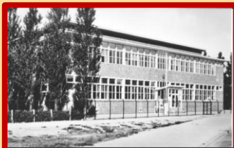
Openbare Lagere School V, later de Prinses Margrietschool
